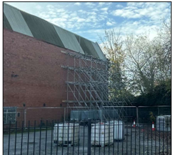
A couple of photos taken on Sunday 11 November showing scaffolding in place to support the end walls of parts of the Arriva (former West Riding) depot and works at Belle Isle, Wakefield.
